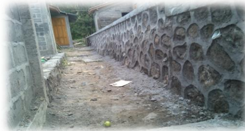
Retaining wall in Umbulharjo Village
