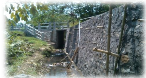
Retaining wall in Sokorini Village
