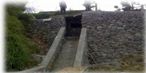
Drainage in Sumber village
